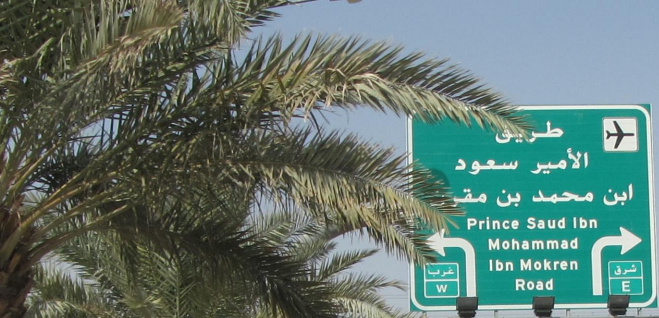
Inappropriate and misleading Direction Sign for roundabout junction – Regulations can specify Format of sign required
